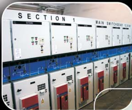
33 kV Switchgear with 1250 A current rating for Al Taif Defence Project (contractor: Al Gihaz) 2010
